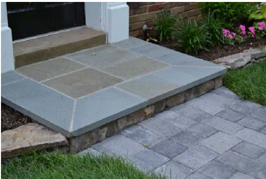
Figure 1 - Sample stoop without stairs
